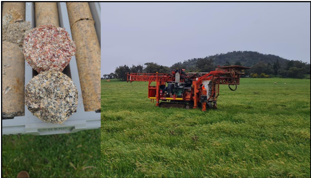
Image one: Examples of weathered granite from GNBDD005, 34 and 40m down hole and right; track mounted diamond drill rig demobilising from the last drill site of the program.
