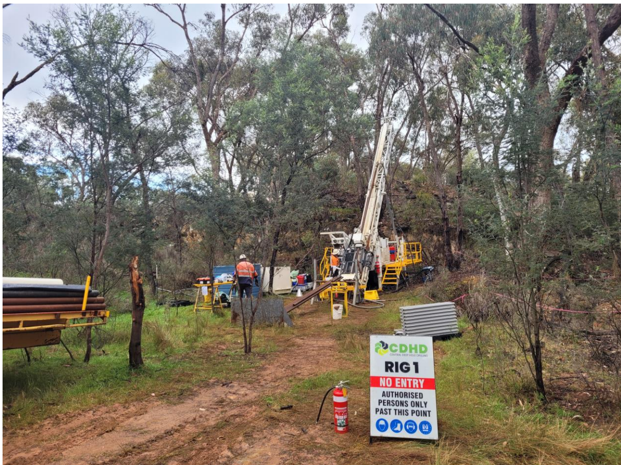
Figure 1: Photo of diamond drill rig on site and drilling at Lewis Ponds
